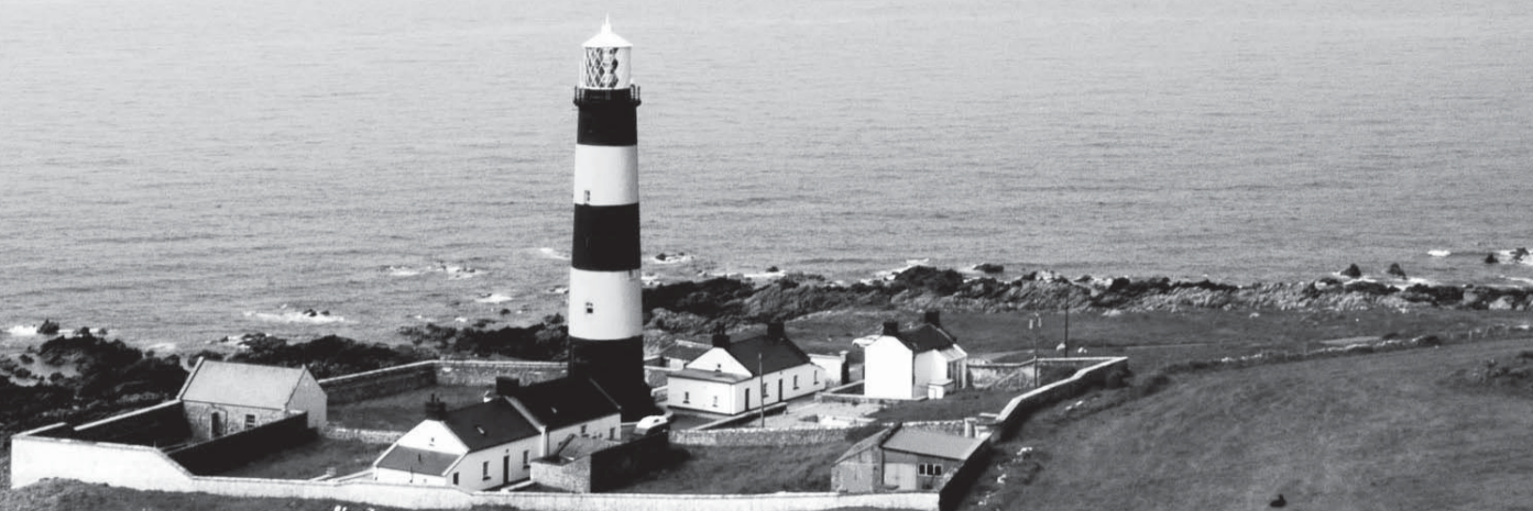
ST. JOHN'S POINT LIGHTHOUSE
